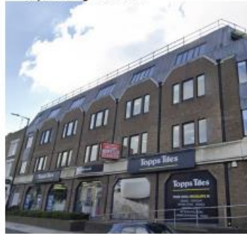
⑤ Facade bay expression, mansard roof
